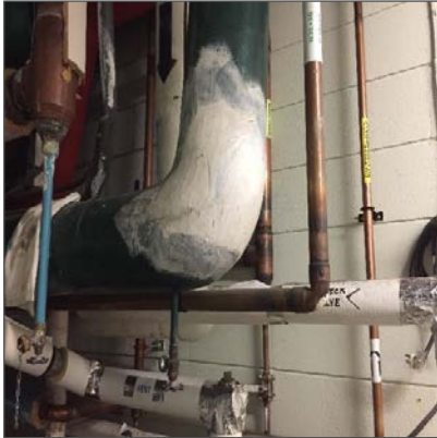
Asbestos-containing parging cement on pipe fitting, Steam Tunnel.
