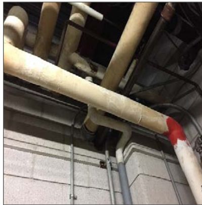
Asbestos-containing paring cement on pipe fittings, Basement Mechanical Room.
