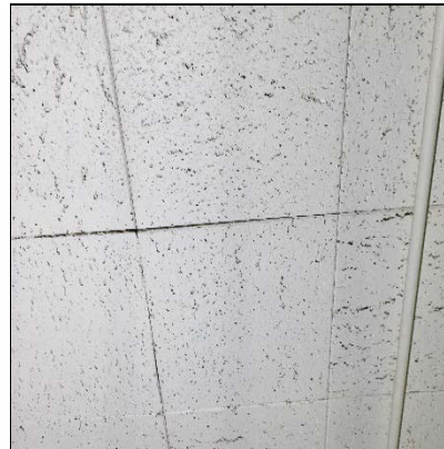
Non-asbestos 12" x 12" glued-on ceiling tiles, random fissure pattern, Basement Room S005 (photo from previous assessment).
