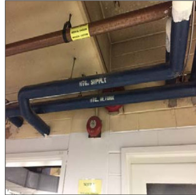
Asbestos-containing parging cement on pipe fittings, Boiler Room.
