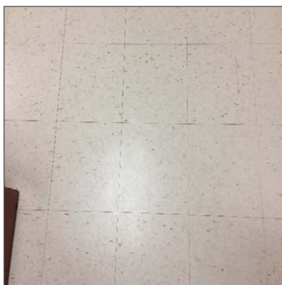
Photo 5 – Non-asbestos 12" x 12" vinyl floor tiles, off-white with multi-colour flecks, Second Floor Corridor.
