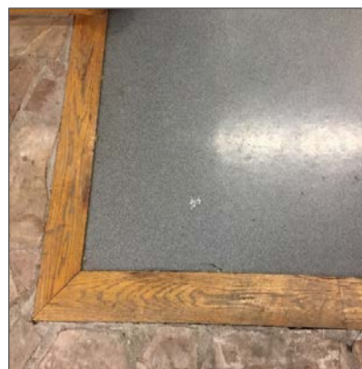
Photo 2 – Non-asbestos vinyl sheet flooring, blue, Level 1 Easy Street Area, East Wing.
