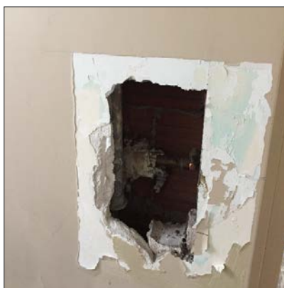
Asbestos-containing Aircell pipe insulation within wall cavity, Level 2 Office Area.
